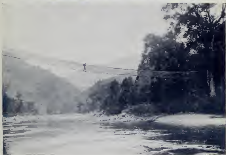
A HAMMOCK BRIDGE AND THE CANE BRIDGE OVER THE NGAWCHANG RIVER.
